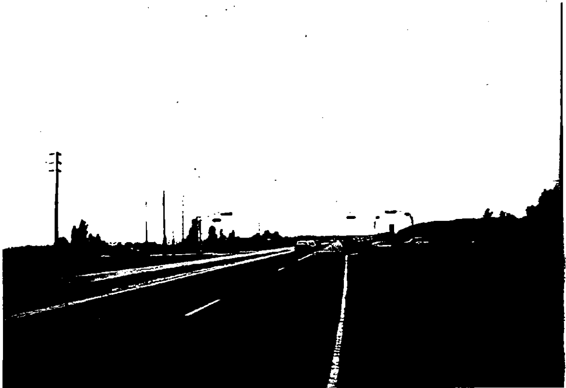
Route I39 & bl. Industriel; direction Nord
